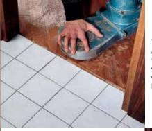
The gap between the two adjacent floors allows for final polishing treatments of wooden or marble surface without damaging the bordering one.
