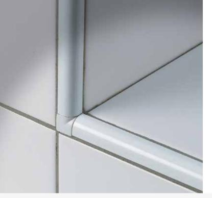
Wall section where the application of the jointing RJI capsule for the profile trim finish is evident.
